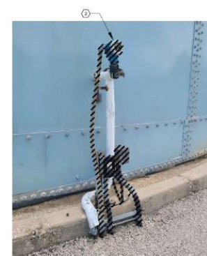
E EXISTING TANK LEVEL INSTRUMENT SCALE: NTS
